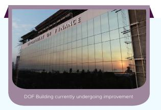
The glass façade reflects an azure landscape designed to minimize pollution and reduce operation costs for the Department. The glass cladding cuts the noise entering the building and also reduces the heat, which makes it energy-efficient.
