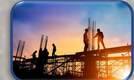
Massive Infrastructure Build-Up
